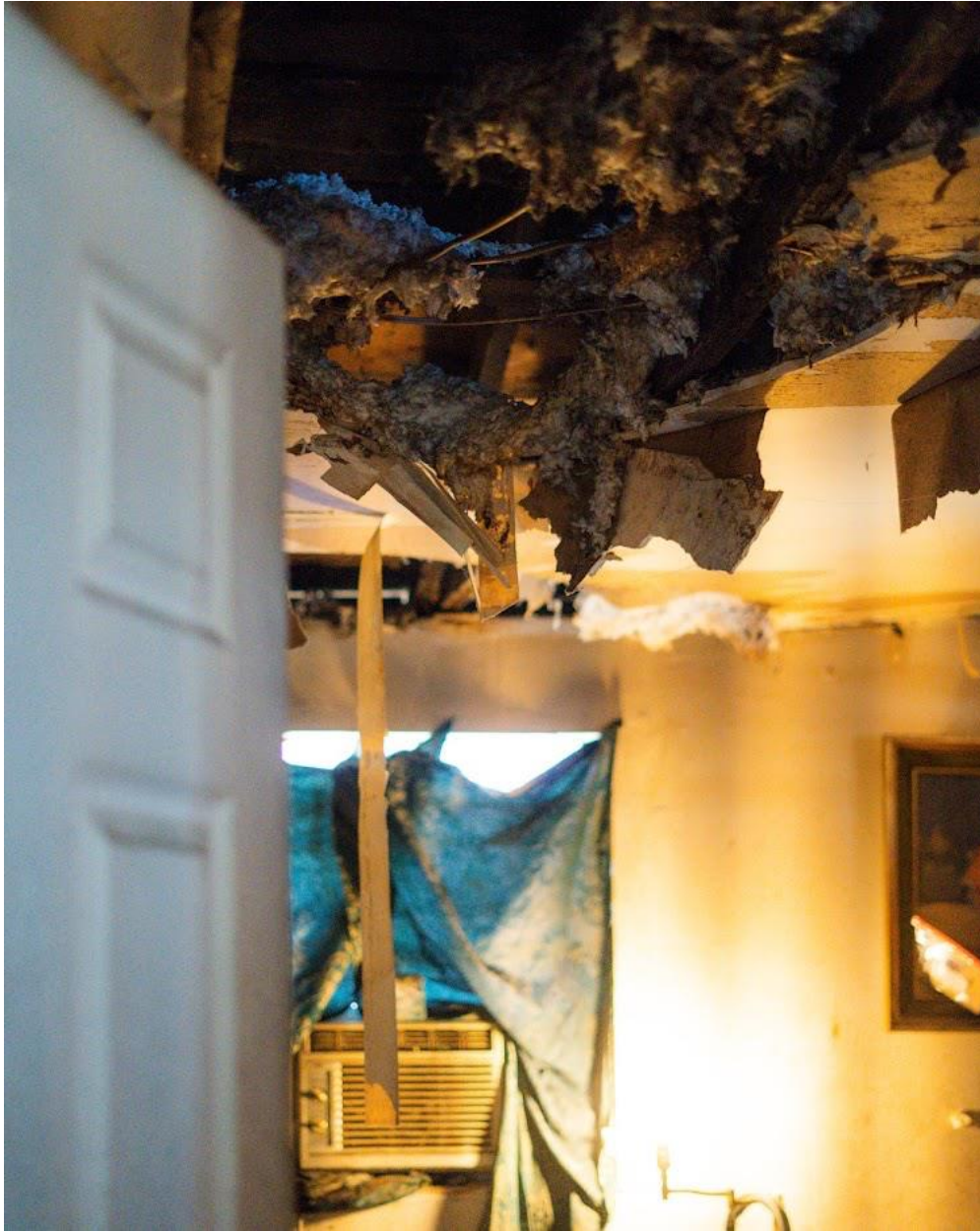
Figure 38. Picture taken by a resident illustrating deficiencies in the roof, and the use of window units in structures that lack insulation.
