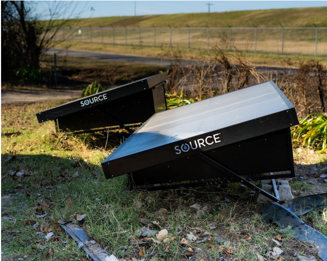
Figure 24. Hydropanels in Springville produce nearly two gallons of drinkable water.
