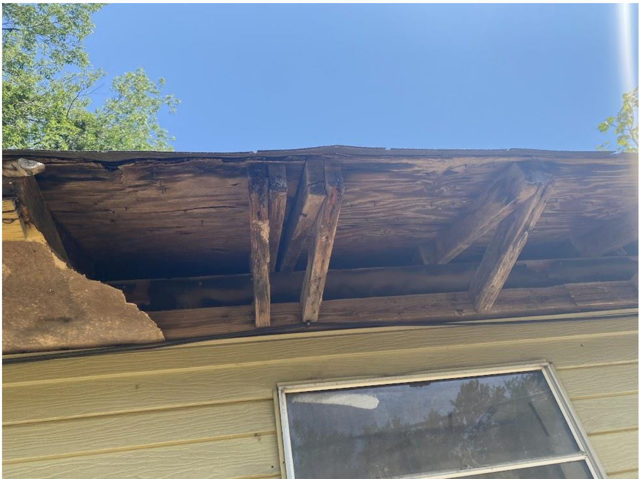
Figure 43. Structural deficiencies in the roofs of aging housing.
